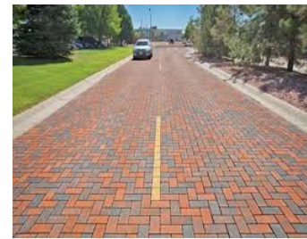
c) Permeable interlocking concrete blocks
